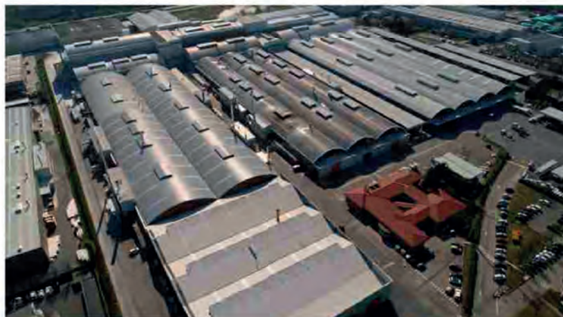
Iris Ceramica Group. Facility Hub
